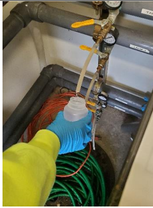
PHOTO 2. SUBJECT: Grab sample collection method at pre-treatment system effluent sampling port, Building 1408. DATE: 21 September 2021. PHOTOGRAPHER: C.J.Lange.
