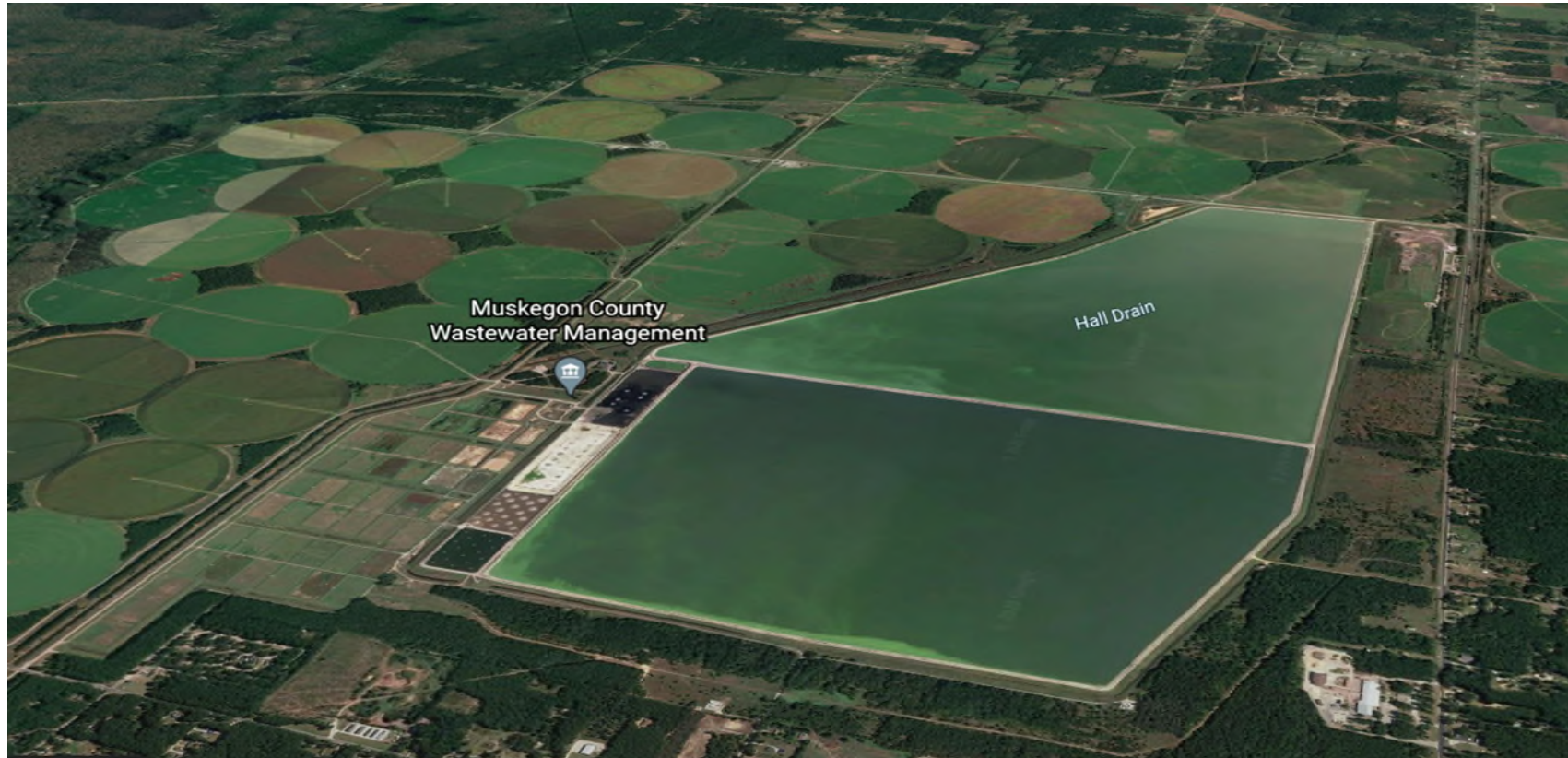
Muskegon County WWMS Metro WWTP storage lagoons, irrigation fields, rapid infiltration beds
