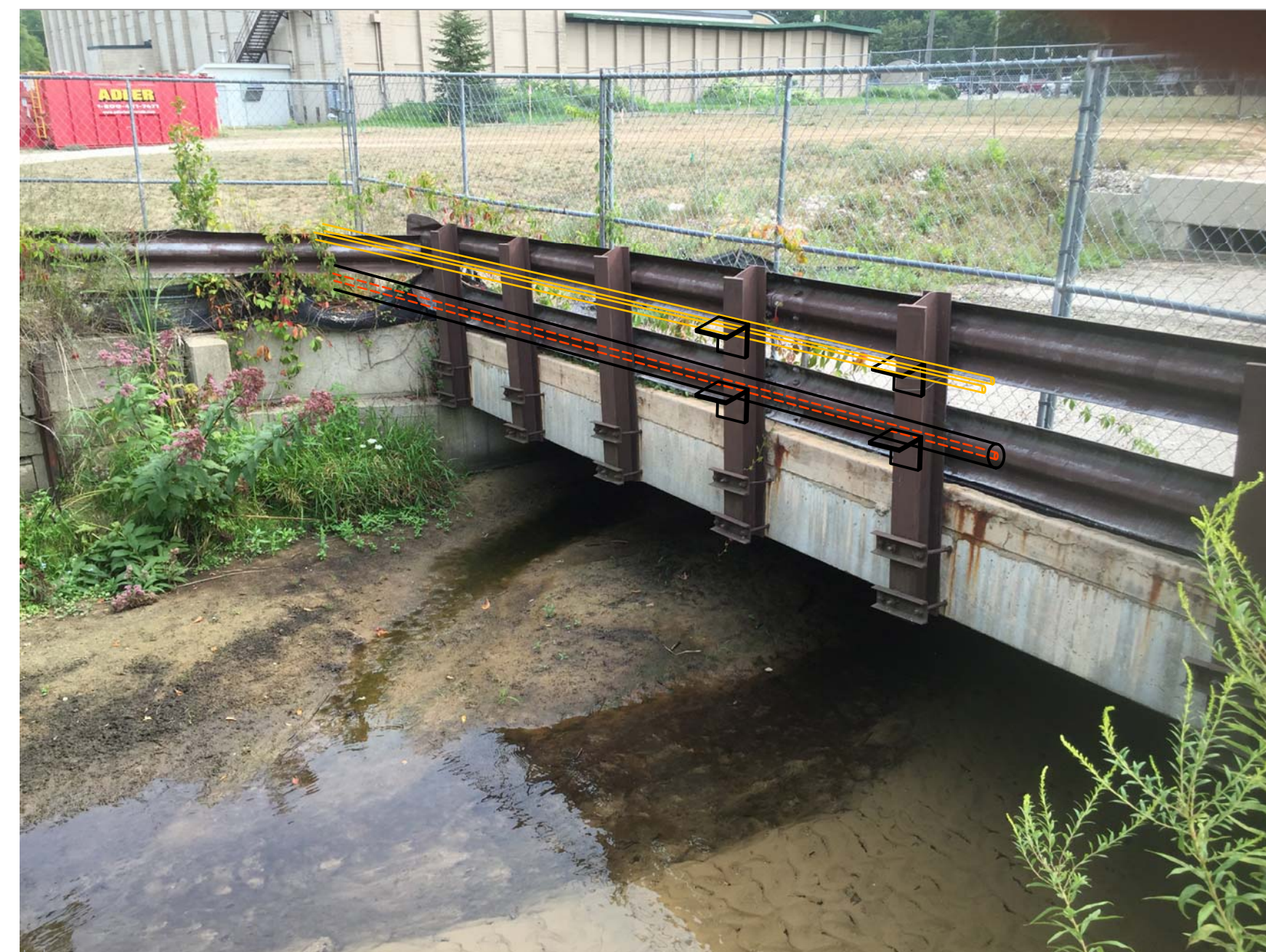
PHOTO AT PIPING DETAIL AT BRIDGE
