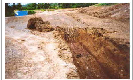
Perimeter Clay Cutoff Wall
