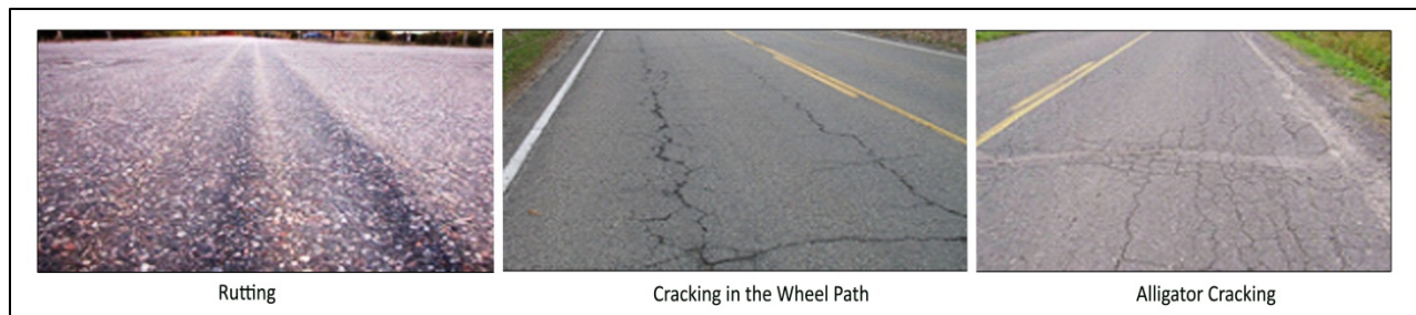
Figure 4: Structural distresses
