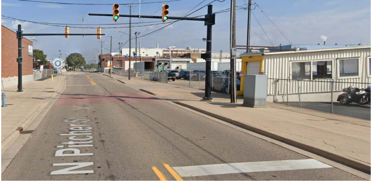
Figure 19: Industrial complex preemption signal
