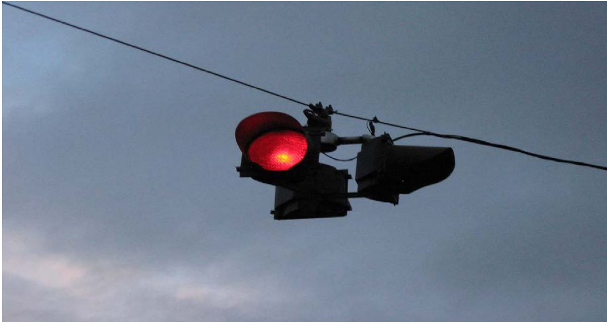
Figure 2: Flashing beacon, which was not considered a traffic signal for the purposes of this study
