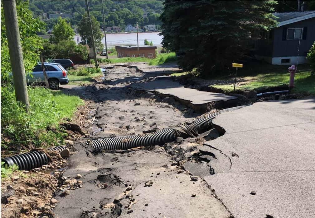
*Figure 2-2: Houghton county culvert failure in Ripley, Michigan*
