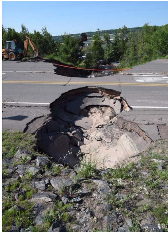
*Figure 2-1: Culvert failure in Houghton, Michigan leading to roadway damage*
