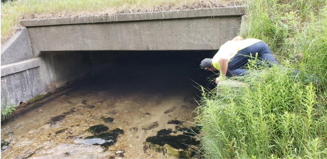
*Figure 4-1: Antrim CRC inspecting a concrete box culvert*
