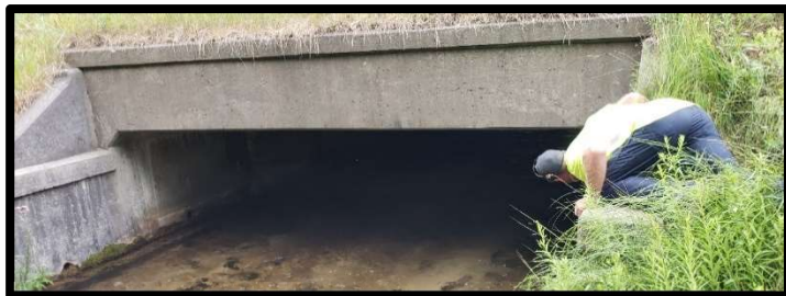
Figure 8: Example of a three-sided box bridge spanning 20 feet or more.
