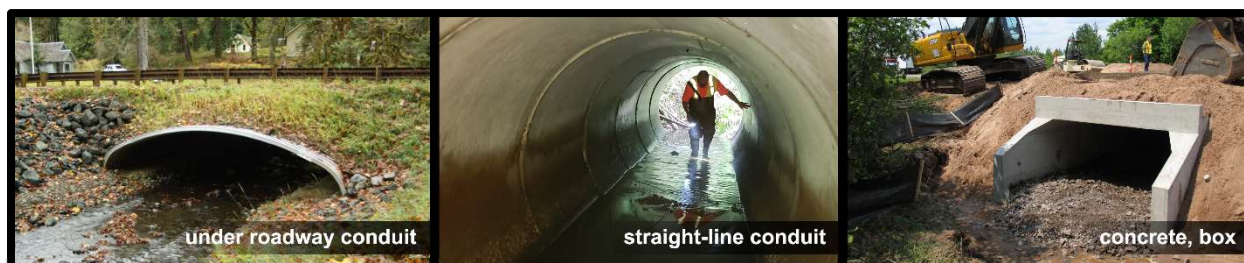
Figure 14: Culverts allow water to pass under the roadway (left), they are straight-line conduits with no immediate drainage structures (middle), and they come in various materials (left: metal; middle and right: concrete) and shapes (left: arch; middle: round; right: box).
