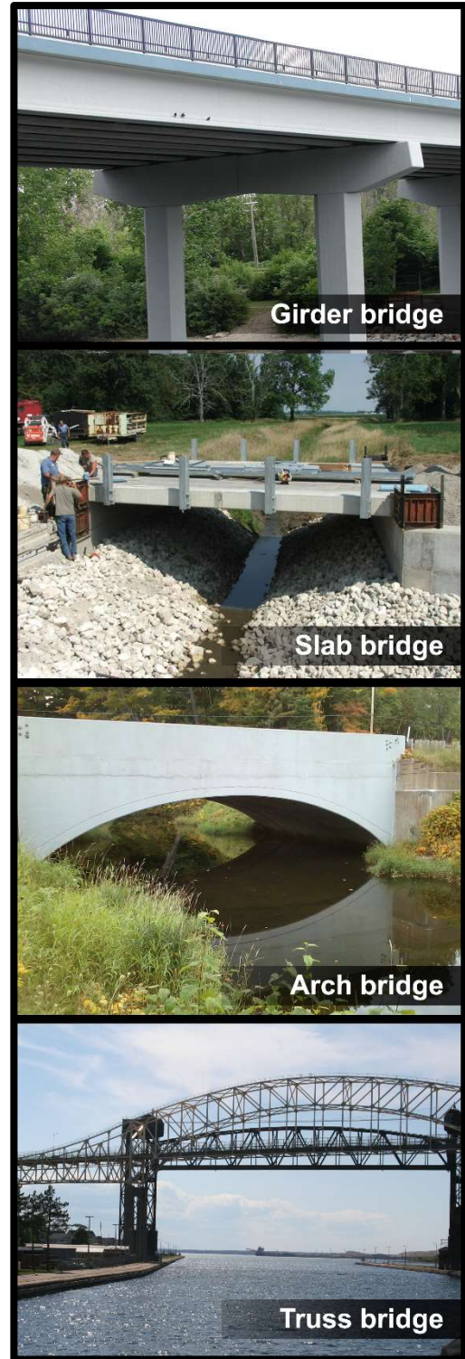
Figure 7: Examples of bridge types in Michigan
