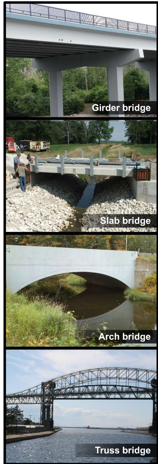
Figure 7: Examples of bridge types in Michigan
