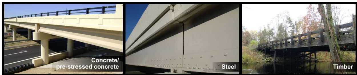
Figure 10: Examples of common bridge construction materials used in Michigan
