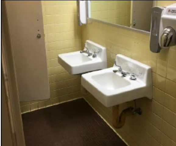
↑ Outdated bathrooms that are not ADA compliant
