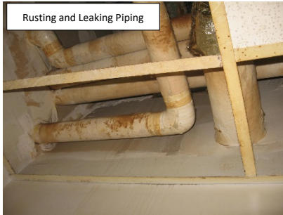
Rusting and Leaking Piping
