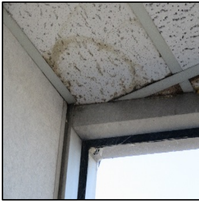
↑ Single pane windows leaking air and water
