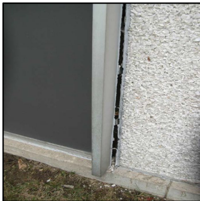
↑ Windows separating from the building
