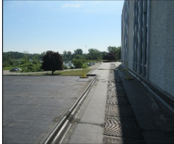
↑ No fall protection in areas of the roof
