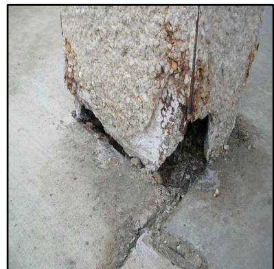
↑ Deteriorating aggregate stucco columns
