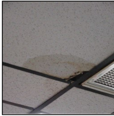
↑ Exterior brick leaks causing water intrusion
