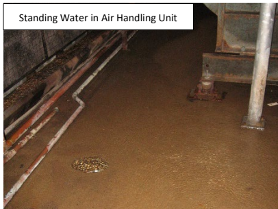
Rusting and Leaking Piping and Pumps
