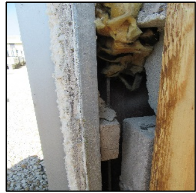
↑ Single pane layered stucco walls. Poorly insulated.
