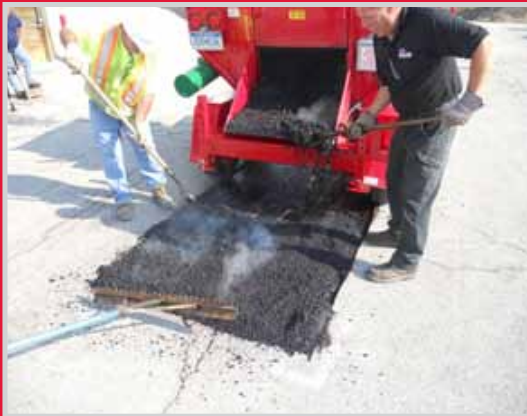
COAT ASPHALT WITH REJUVENATOR
