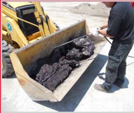
COAT ASPHALT WITH REJUVENATOR
