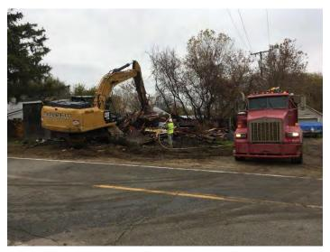
Based on the results of the remedial investigation, DLZ recommended that the building be demolished as impacted soils were remaining under the building. DLZ prepared bid specifications for the abatement of all asbestos containing materials, the removal of all hazardous materials, the demolition of the building, removal of contaminated soil, backfill compaction of sand, and the restoration of the site with topsoil and seed. DLZ reviewed all bids on behalf of EGLE and made the
