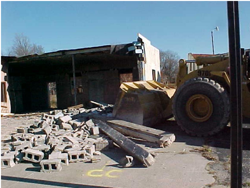
PHOTO 3 (22 NOV 04): SEGREGATION OF CONCRETE AND STRUCTURAL STEEL FOR SALVAGE FROM THE SOMERS MOBIL BUILDING DEMOLITION.
