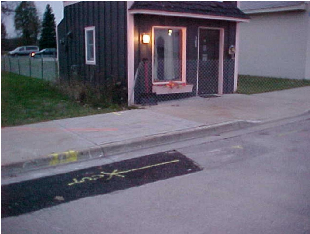
PHOTO 5 (22 NOV 04): LOOKING NORTHWEST AT NATURAL GAS LINE CUT POINT, WHICH IS TOO FAR TO THE SOUTH AND WILL INTERFERE WITH THE SHEET PILING INSTALLATION.
