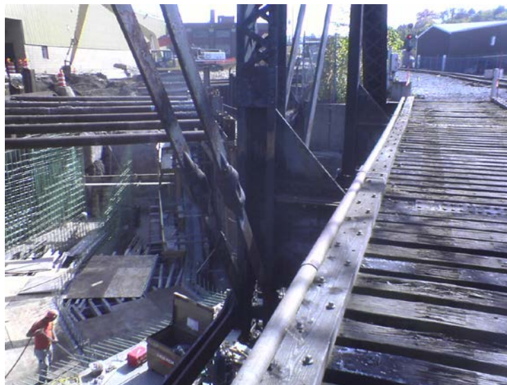
CSO Earth Retention System and Tunnel
