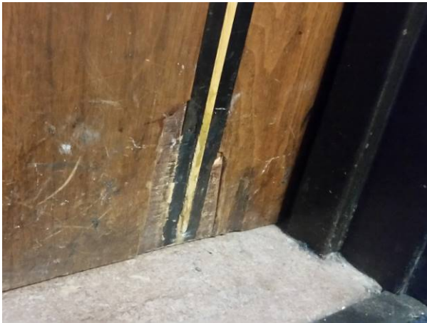
Photo 7: Damage to wood door veneer
