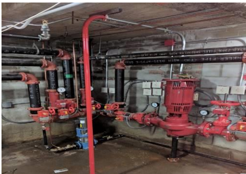
Photo 4: Fire Sprinkler Riser
