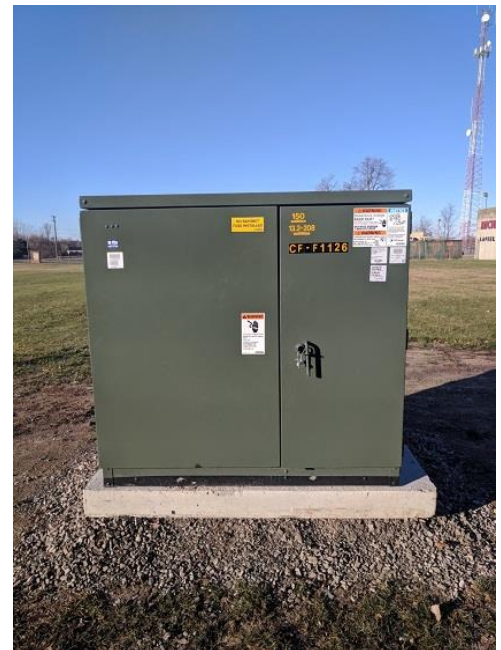
New Electrical Transformer
