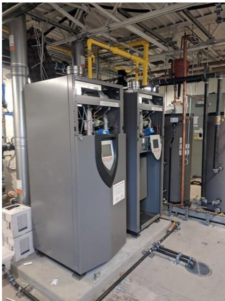
Size: Boilers and Electrical Equipment; 19,500 sq.ft. Roof Estimated Cost of Construction: $834,000
