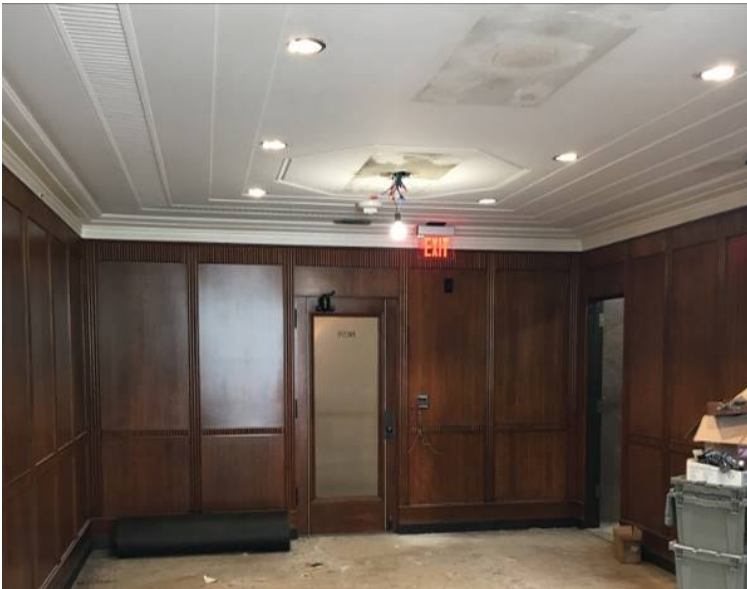
Photo 5: Walnut wall panels restored in the Library.
