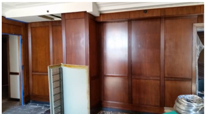
Photo 9: Bookcases in Judge's Office prior to restoration. Photo 10: Repair needed where bookcases were removed. Photo 11: Wood wall panels restored in Judge's Office.
