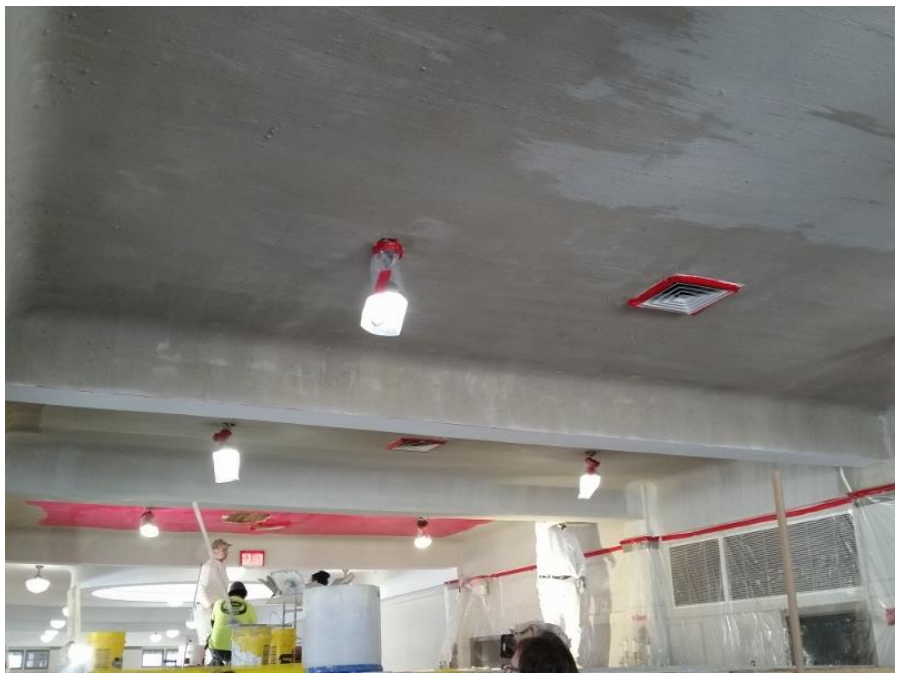
Photo 2: Plaster Repair
