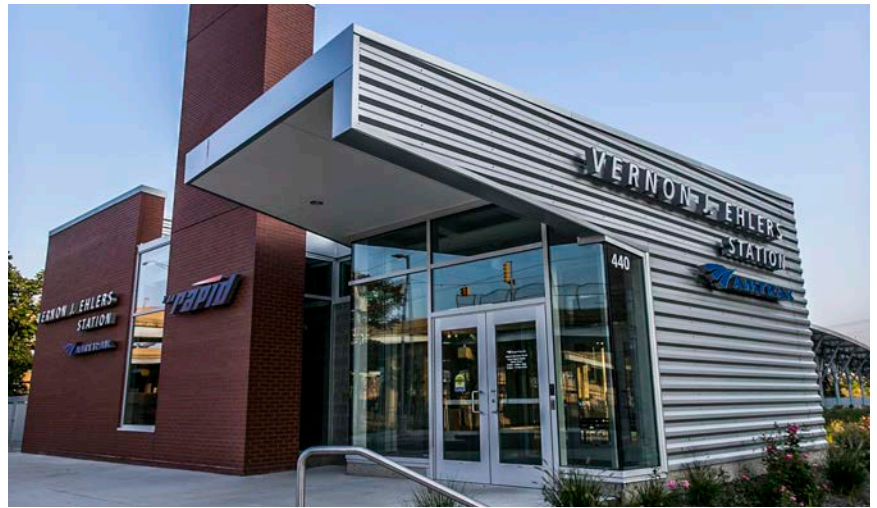
AMTRAK - "The Rapid" Passenger Station Relocation | Grand Rapids, MI
