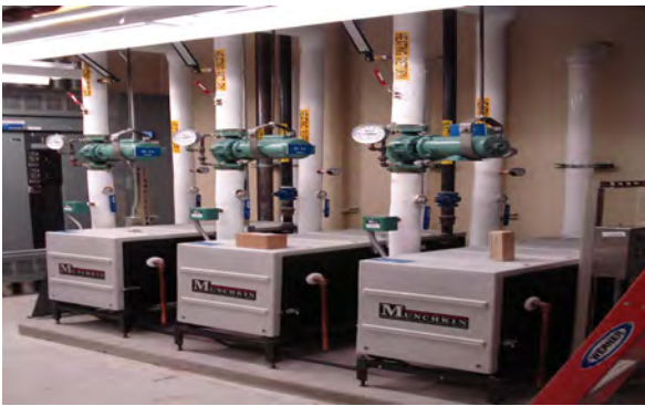
Boiler system for in-floor radiant heat and snow-melt
