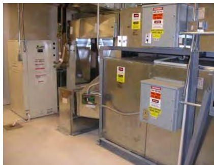
Energy recovery units with Geothermal heating system
