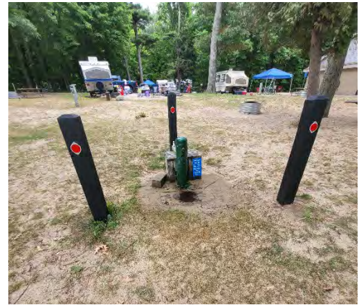
This existing jug filler is not ADA compliant and required replacement to meet ADA requirements
