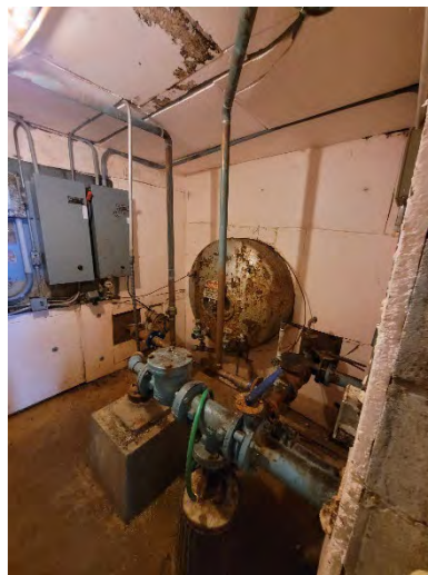
The existing water distribution system should be evaluated to replace existing pump motors with a VFD system to accommodate better system pressures and water reliability. Additionally, wells should be evaluated for new controls that will bring efficiencies to the water system.
