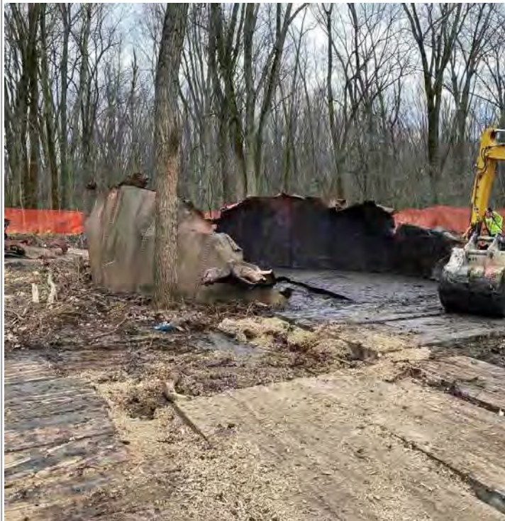
Caption: AST after sludge removal
