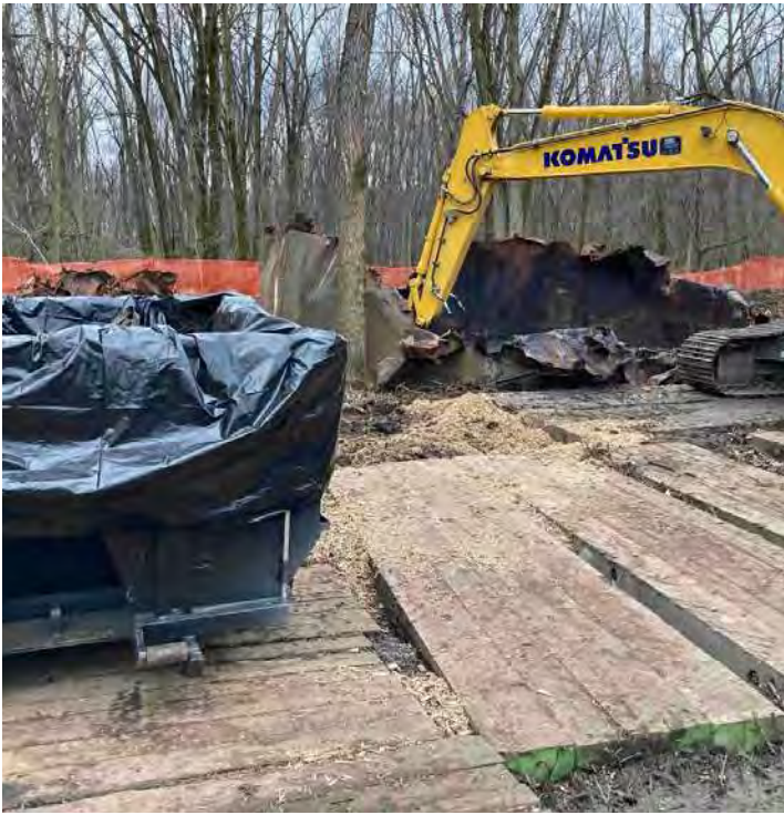
Caption: Sludge removal from AST
