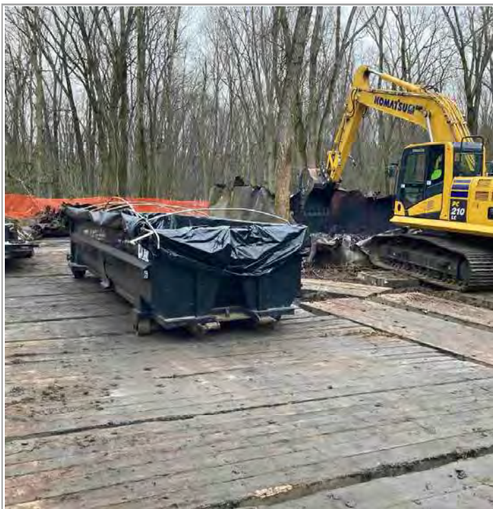
Caption: Sludge preparation for solidification
