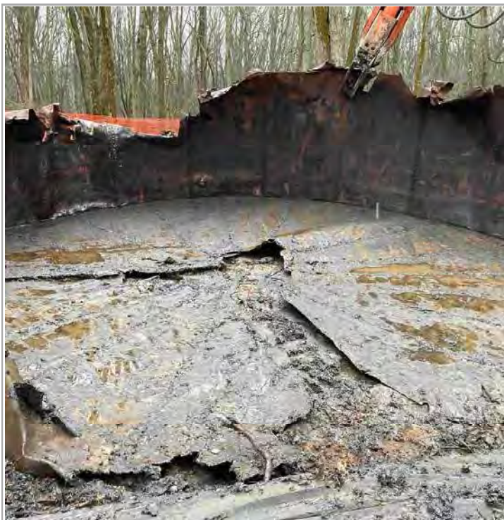
Caption: Removal/demolition of AST
