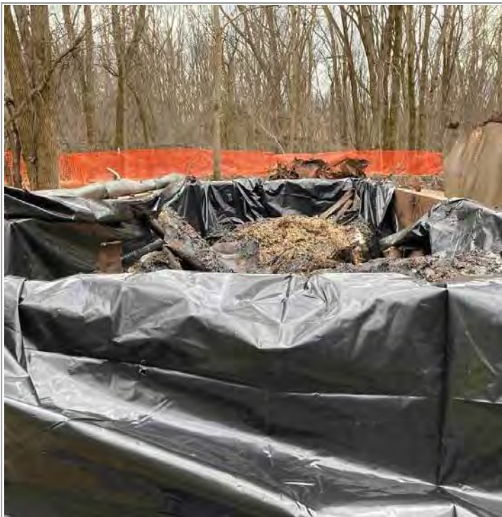
Caption: Removed solidified sludge materials
