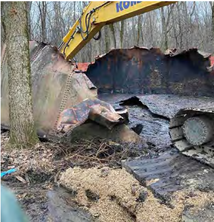
Caption: Sludge removal from AST
