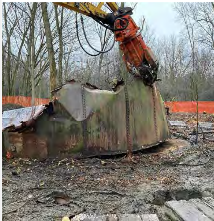
Caption: Removal/demolition of AST
