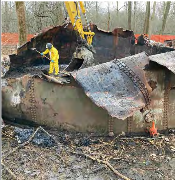
Caption: Sludge removal from AST
