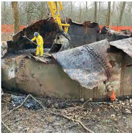
AST dismantling and cleaning.
