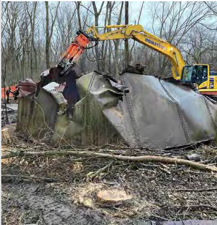
Caption: Removal/demolition of AST
