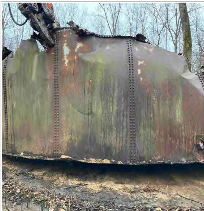
Caption: Removal/demolition of AST
