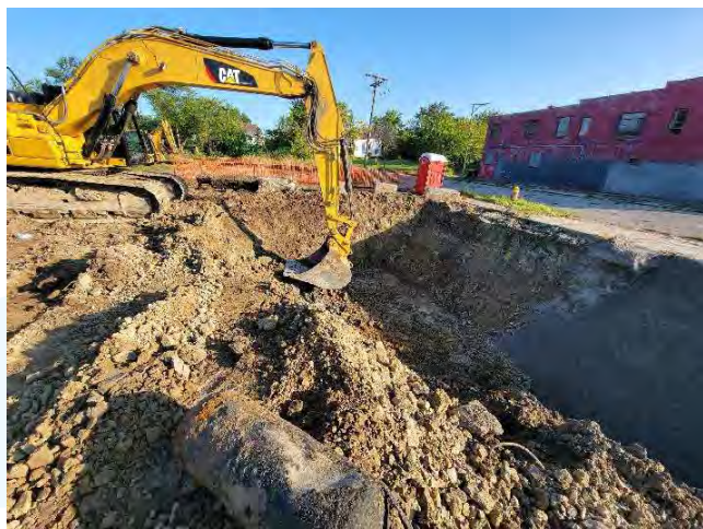
Excavation of USTs and impacted soil at a former gas station.
