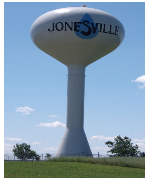
Village of Jonesville Water Tower
