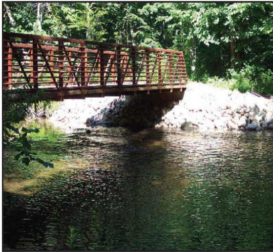
Ionia Recreation Area Pedestrian Bridge
