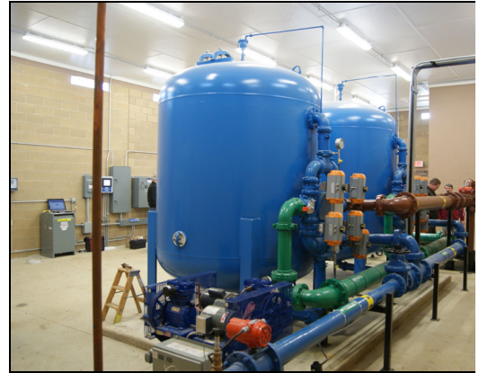
Waldron Well House and Iron Removal Equipment
