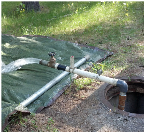
Northern Wells Pump Test at Hartrick Pines
