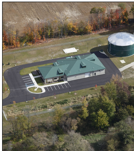
Mason Water Treatment Plant
