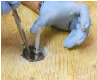
Figure 6. Seal annular space
