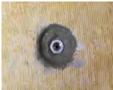
Figure 7. Seal complete
