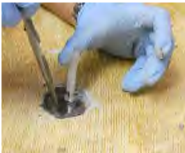
Figure 6. Seal annular space
