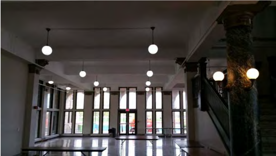
Photo 3: Sprinkler installation on the first floor
