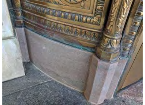
Picture 10: After Stone Repairs
