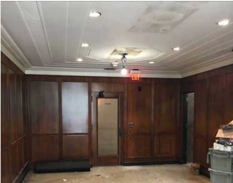
Photo 5: Walnut wall panels restored in the Library.
