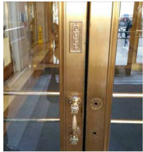
Picture 5: Missing original brass hardware was replicated for the new doors
