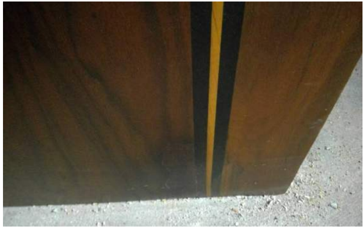
Photo 8: Wood veneer repaired on door and door refinished.
