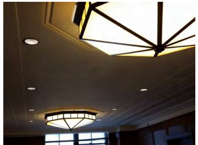
Photo 6: New custom light fixtures in Library.
