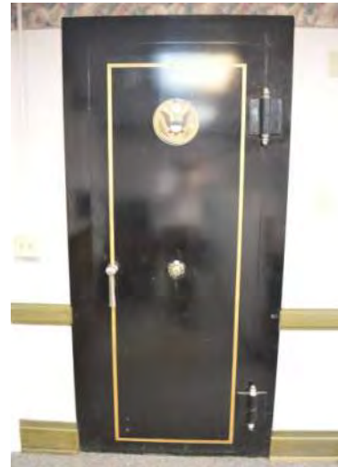
Photo 3: Original vault door.
