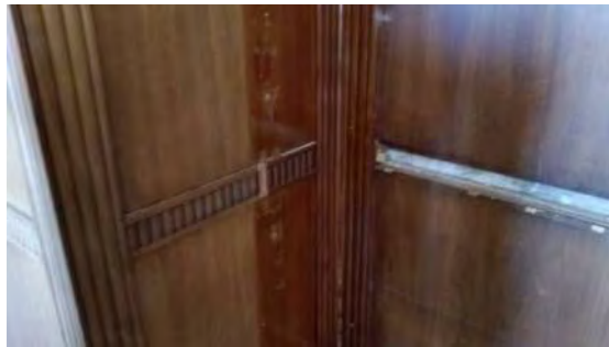
Photo 8: Wood veneer repaired on door and door refinished.
