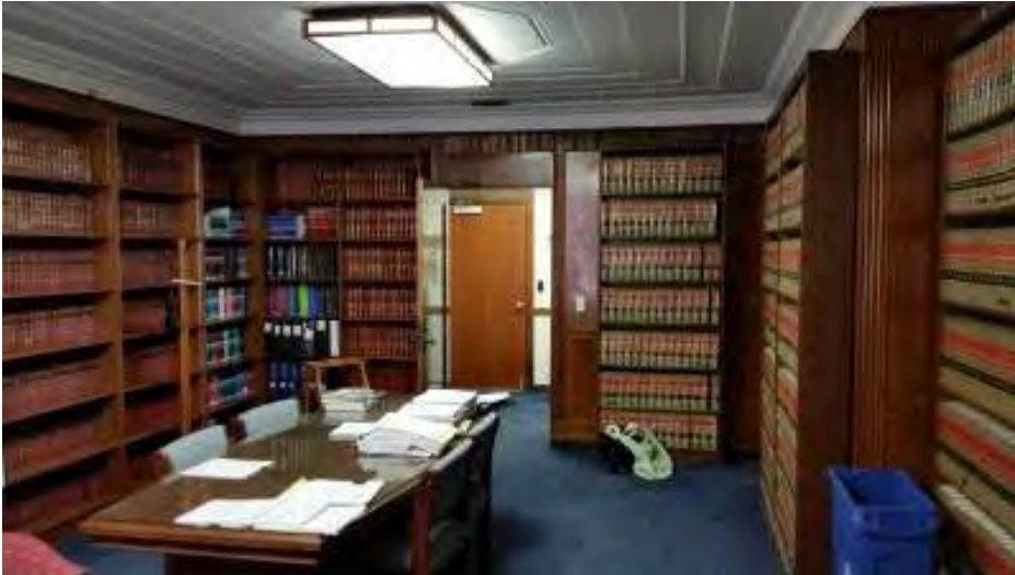
Photo 3: Library prior to restoration with bookcases attached to original wood Panels and surface mounted fluorescent lights.
