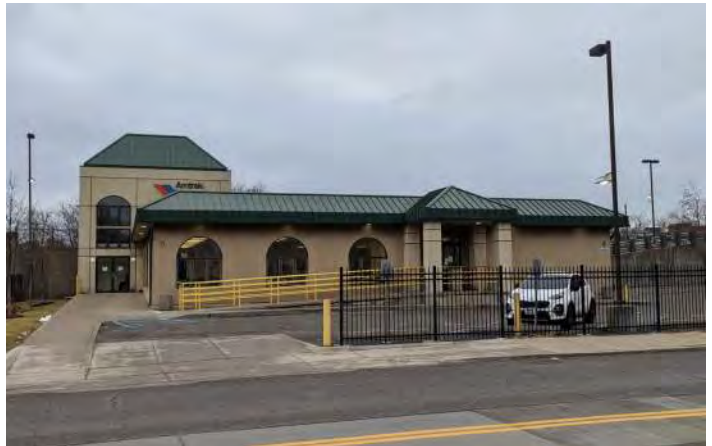
Photo 1: Amtrak Station Detroit Terminal
