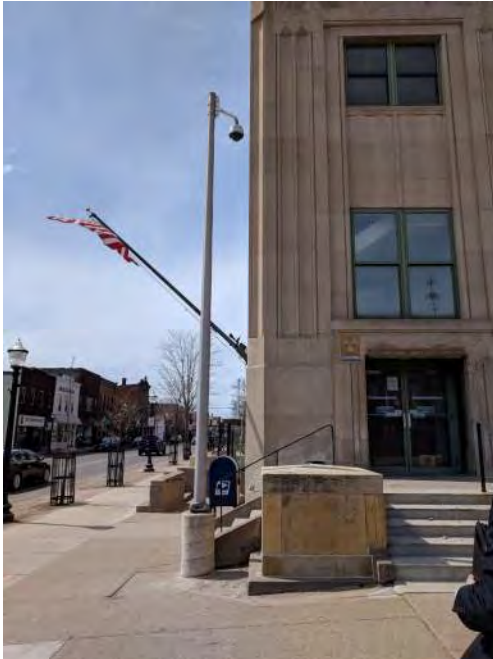
Photo 1: Bollards and Flagpole Before
