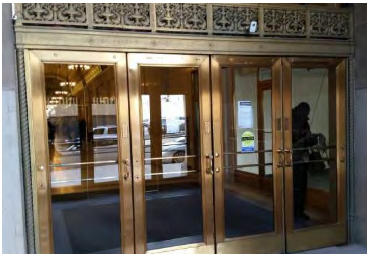
Picture 4: Interior view of the Cass Avenue (East) entrance before renovation
