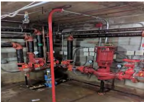
Photo 4: Fire Sprinkler Riser
