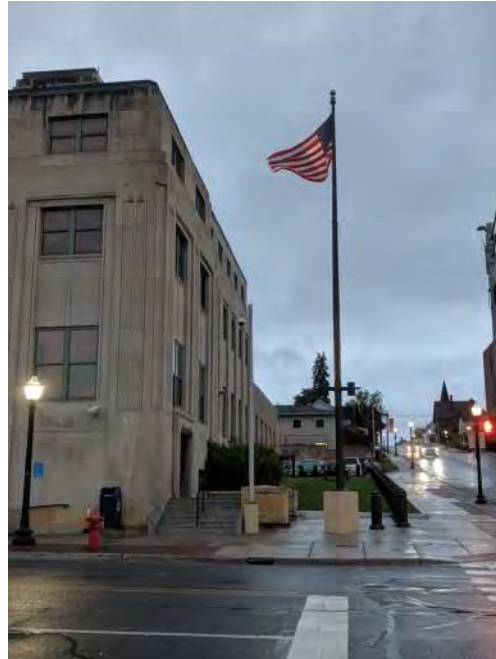
Photo 2: Bollards and Flagpole After
