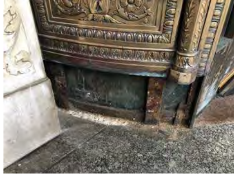
Picture 9: During Stone Repairs
