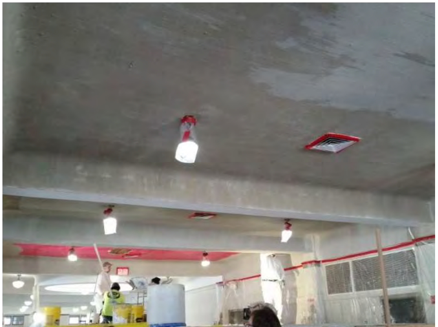
Photo 2: Plaster Repair
