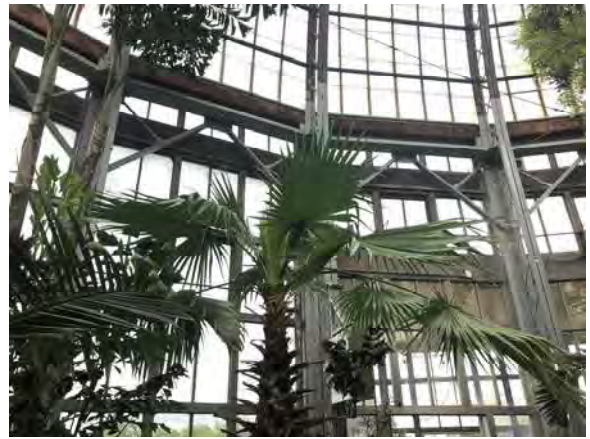
Picture 4: Conservatory Repaired
