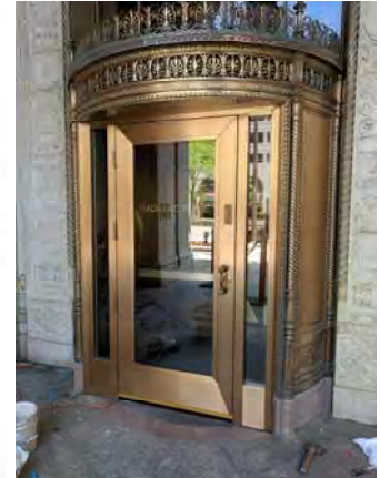
Picture 2: New exterior door
