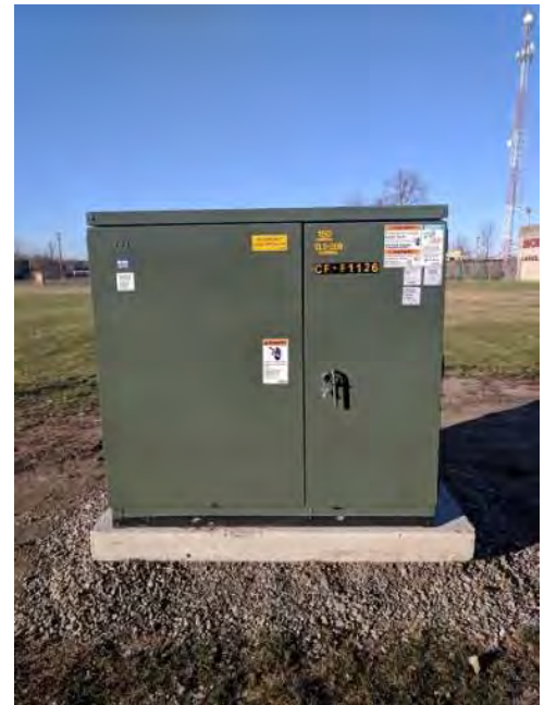
New Electrical Transformer
