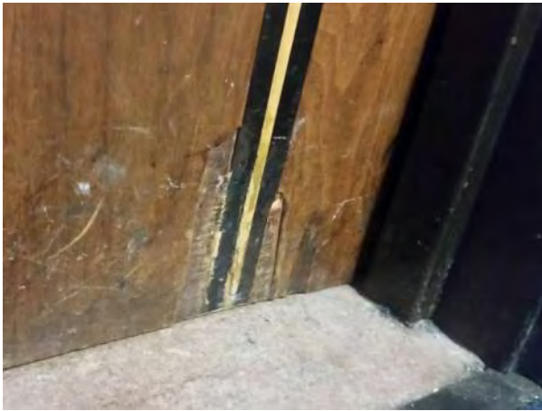
Photo 7: Damage to wood door veneer
