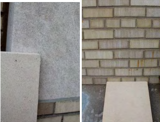
Photos 4 & 5: Samples of the concrete panels in front of the building.
