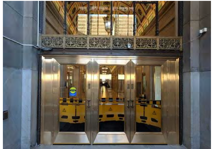
Picture 7: Cass Avenue entrance after renovation
