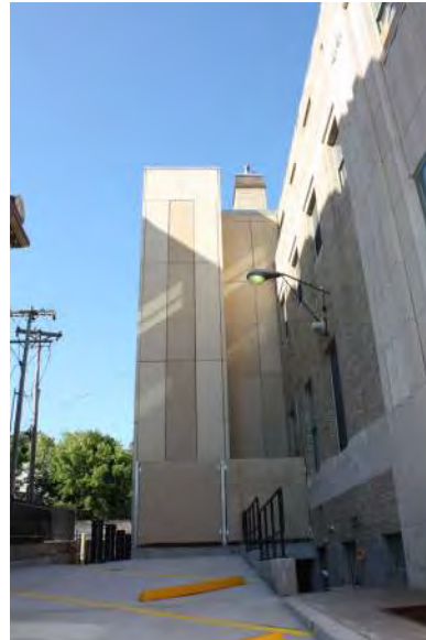
Photo 2: Elevator Tower Addition.
