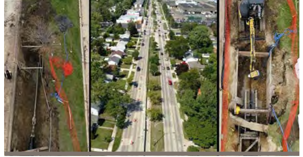
Award-Winning 16-Inch Transmission Main Rehabilitation
