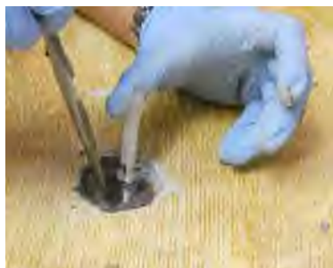
Figure 6. Seal annular space
