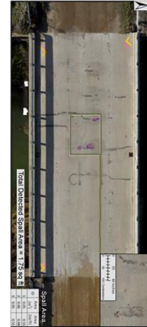
Detected Spalls
