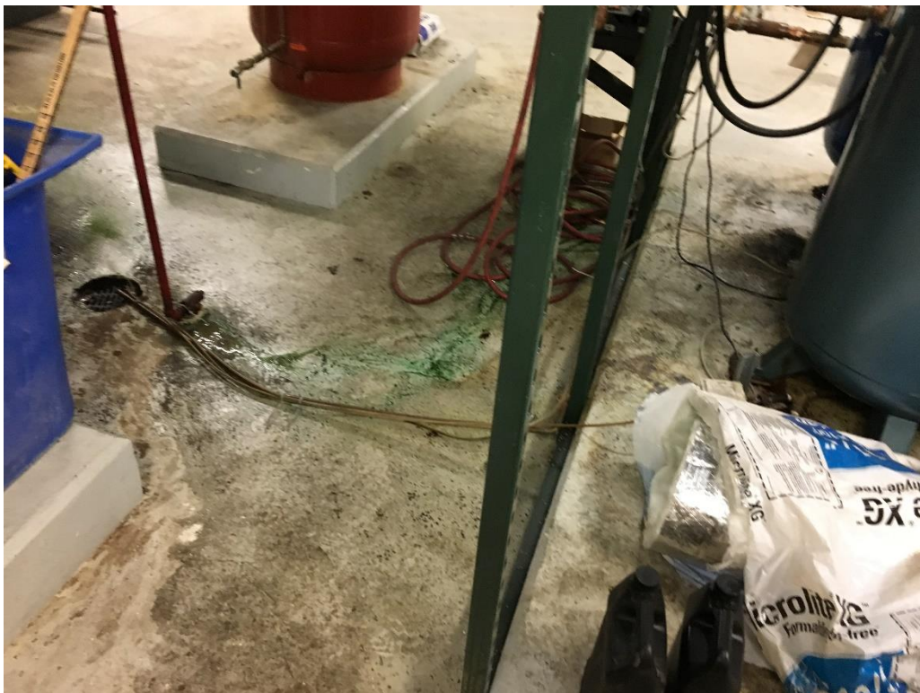
Green fluid migrating towards drain from Hankison air drying unit
