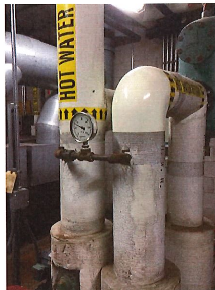
Description: Visible Mold on Insulation in Mechanical Room
