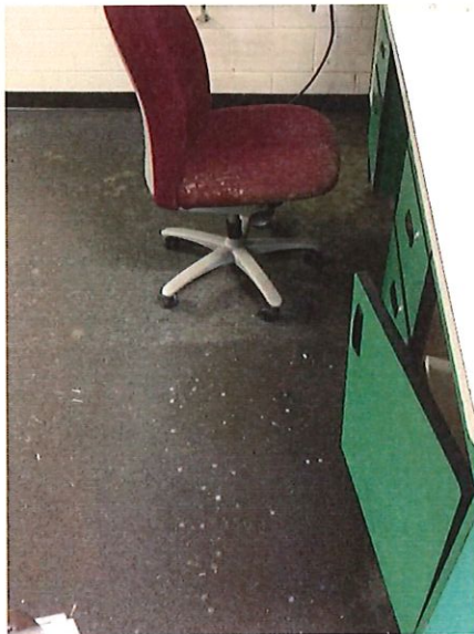
Description: Visible Mold in Office
