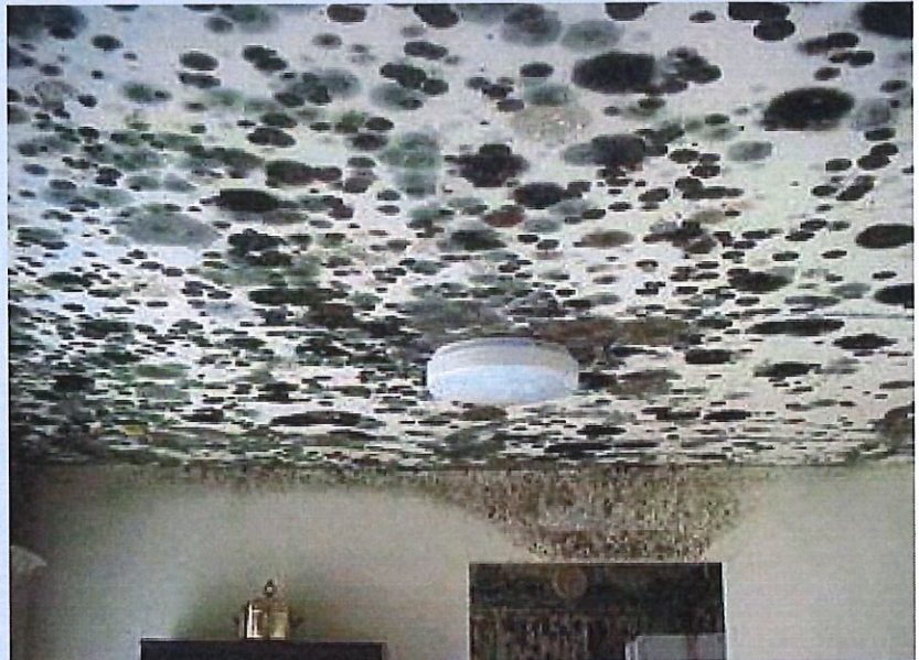
Photo 2: Extensive mold contamination of ceiling and walls
