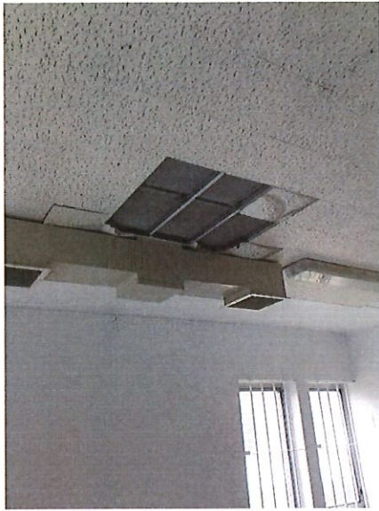
Description: Historical Water Damage in Visiting Area Date: 10/10/2018 Taken By: AGK
