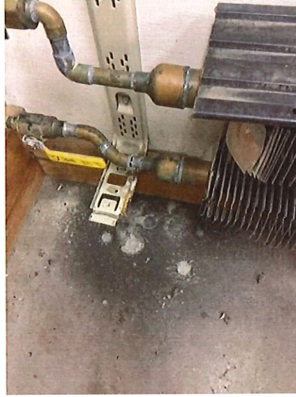
Description: Example of Mechanical System Drainage seen Throughout Date: 10/10/2018 Taken By: AGK
