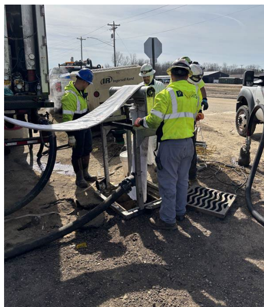
Epoxy liner being installed in a storm sewer.
