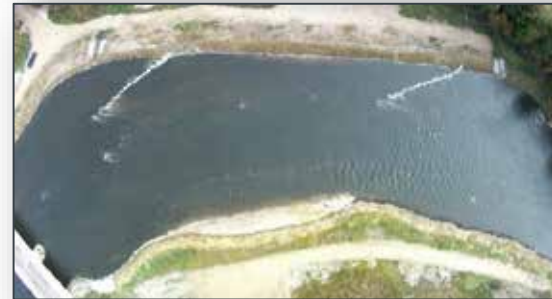
Aerial view after J-hook Installation
