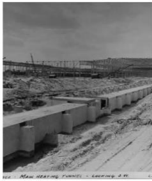
HEATING TUNNEL - LOOKING S.W.
