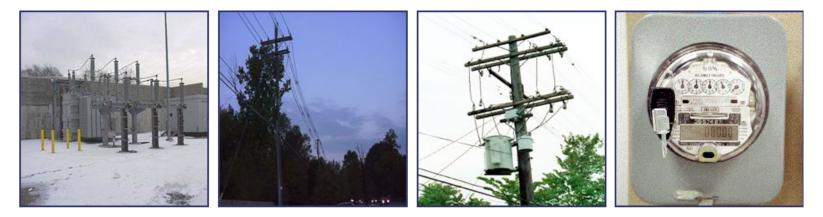
Substation: Steps down voltage for distribution Distribution Lines: Lower voltage lines distribute power from substations to the end customer
