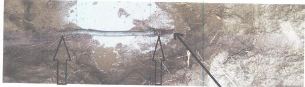
This is the City Side and it is made of lead piping.
