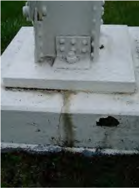
(2) Delaminated coating on leg foundation, and missing grout beneath baseplate.
