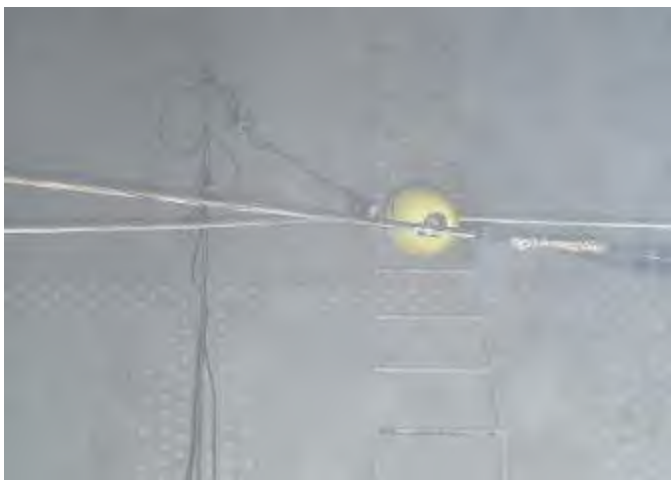
(30) Sidewall/bowl ladder, and cathodic protection float.
