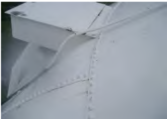
(26) Overflow weir box and antenna cable showing rusting.
