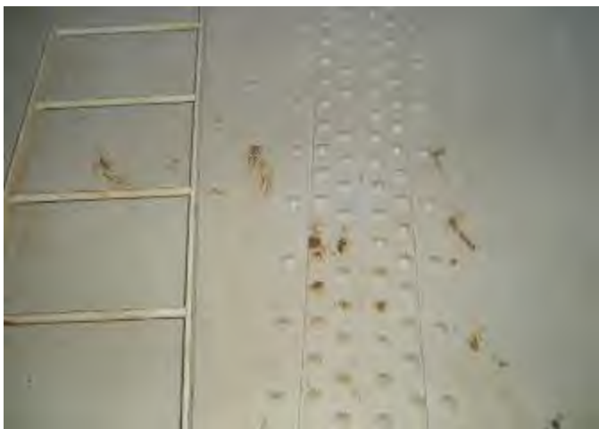
(32) Coating breaks on lower sidewall rivets.
