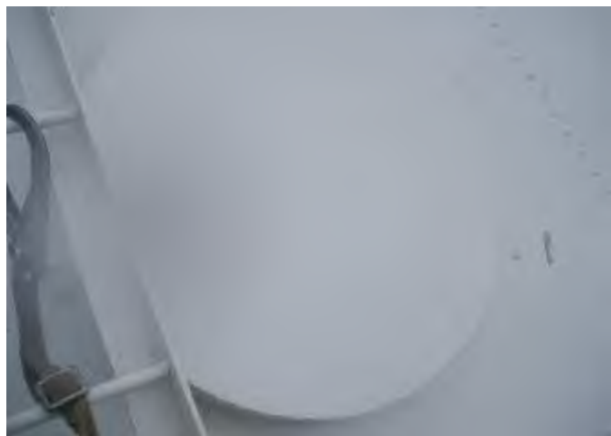
(25) Roof ladder over top of the roof manway.
