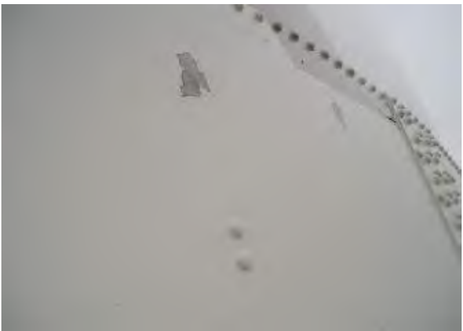
(17) Delaminated topcoat on sidewall.
