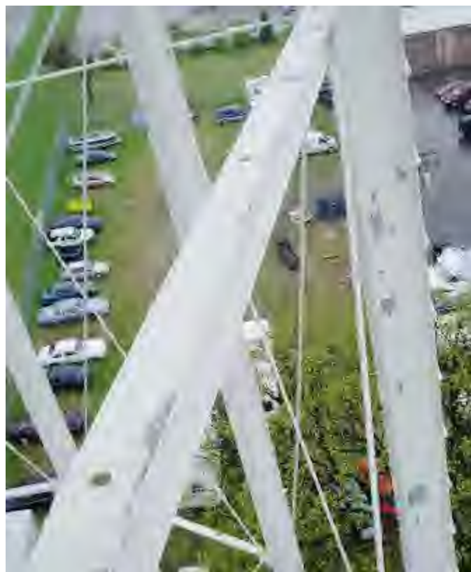
(9) Delaminated topcoat on strut and leg.
