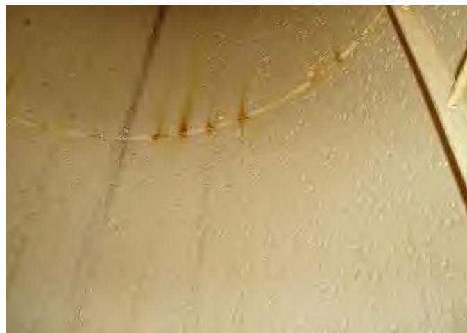
(43) Rust staining at riser can stitch welds.
