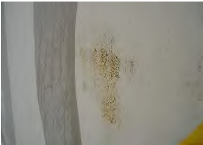
(20) Pinhole rusting on sidewall.
