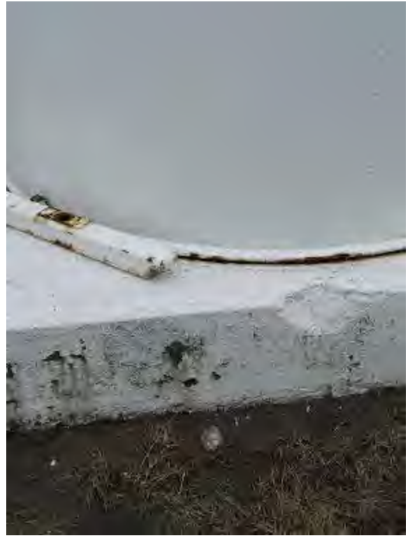
(3) Missing grouting on riser baseplate, and delaminated coating on foundation.
