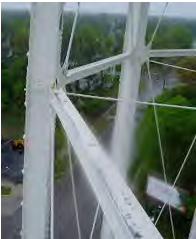
(8) Rust at buckles, and delaminated topcoat on strut.
