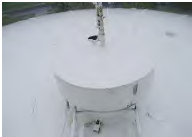
(27) Roof vent with antenna mount and open hole.
