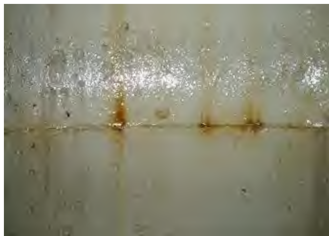
(41) Rust staining at riser can stitch welds.
