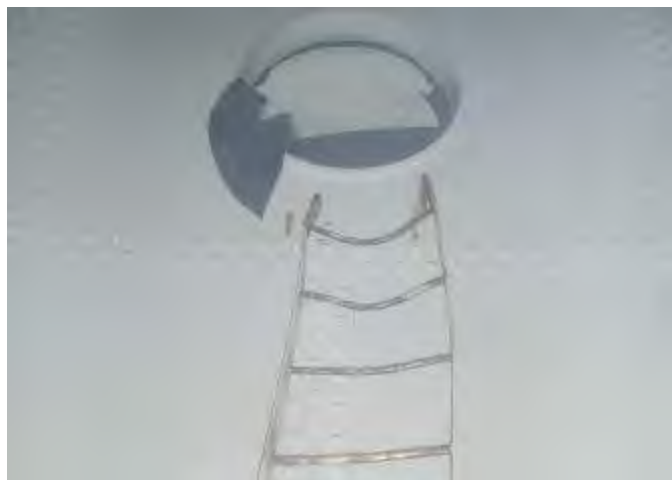
(31) Damaged 4 ft. of sidewall/bowl ladder, and torn gasket.
