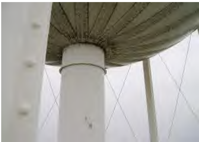
(12) Delaminated coating on riser, and algae on bowl.
