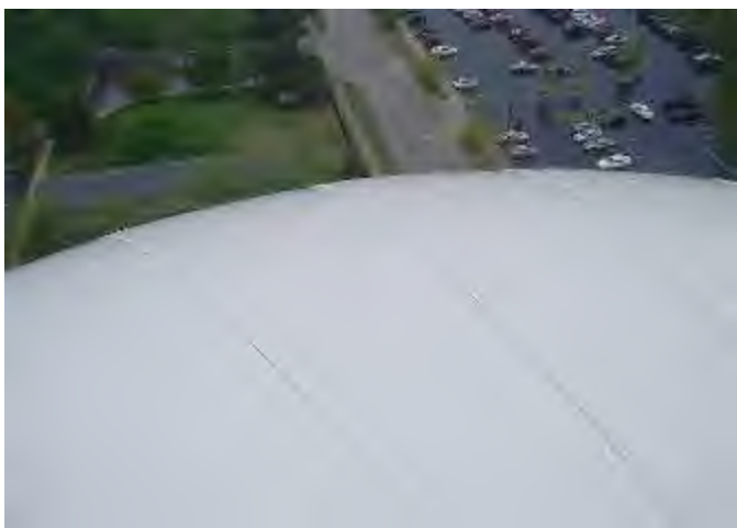
(22) Exterior roof coating is intact.
