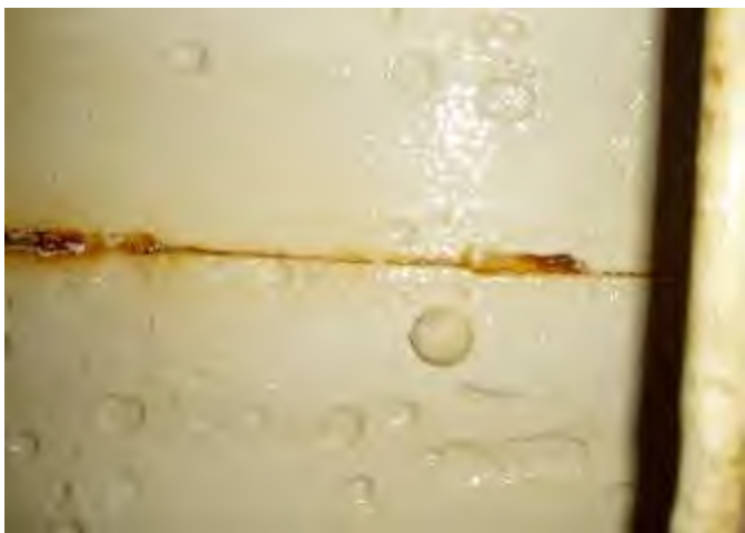
(42) Rust staining at riser can stitch welds.
