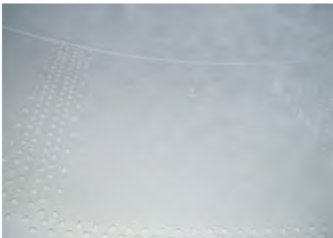
(36) Coating intact on previous pitting.
