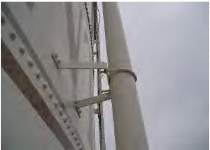
(19) Faded lettering, and overflow bracket.
