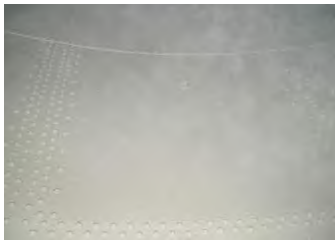
(35) Coating intact on sidewall.
