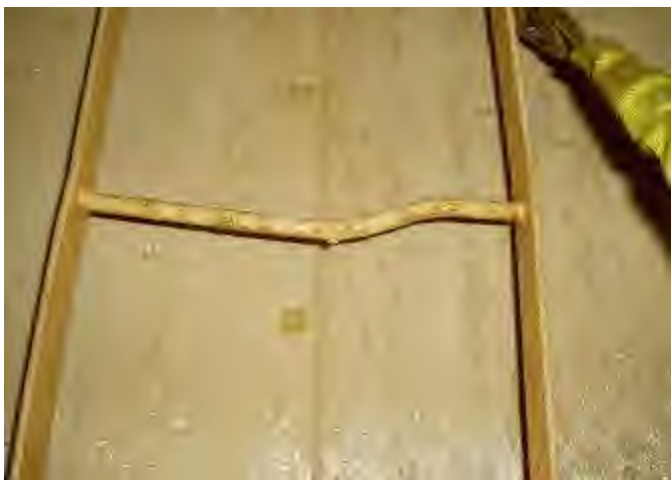
(50) Deformed riser ladder rung.
