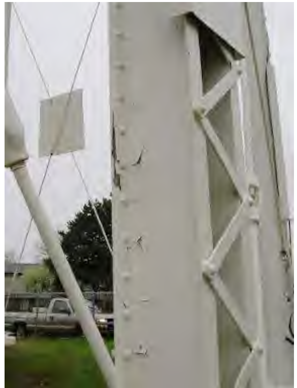
(5) Delaminated topcoat on lattice leg.
