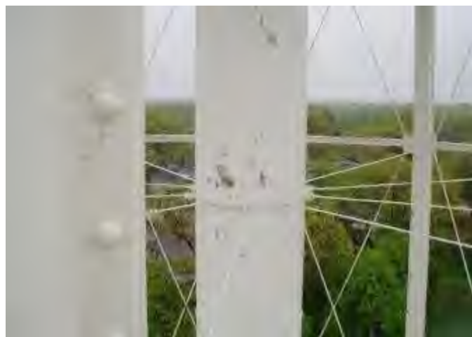
(11) Delaminated coating on riser, and rust staining.
