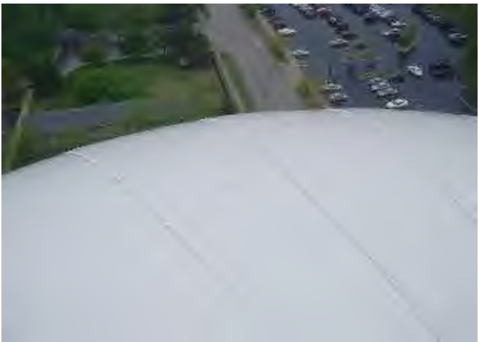
(21) Roof coating is intact - areas of bleed-through.
