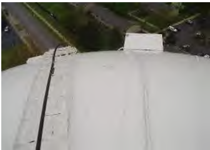
(24) Roof ladder over top of the roof manway.
