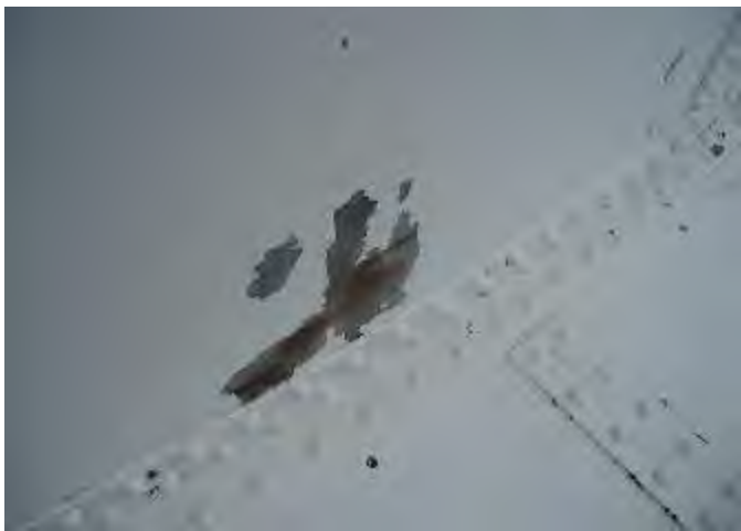
(16) Delaminated coating/rust at balcony.
