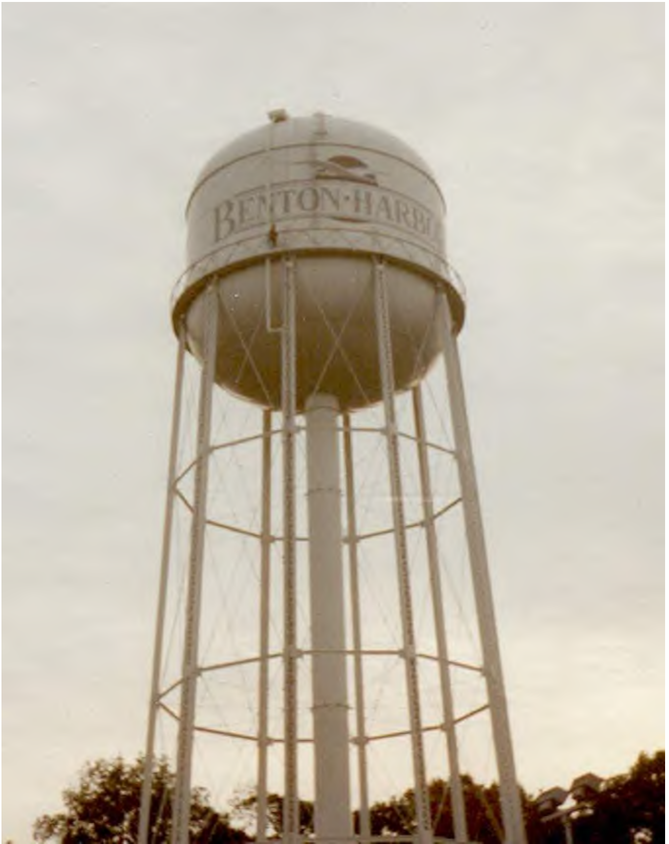
(1) Benton Harbor 650,000 gallon water storage tank.
