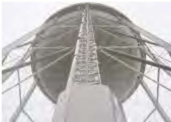
(49) Leg ladder fall prevention rail and vandal guard.
