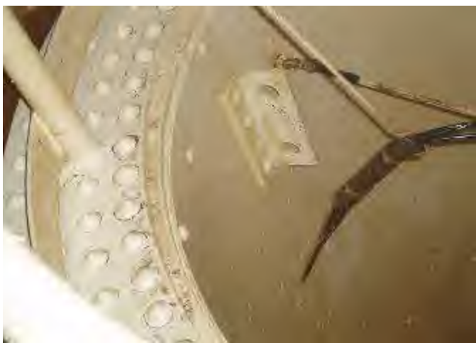
(40) Riser-to-bowl junction - coating protecting steel.
