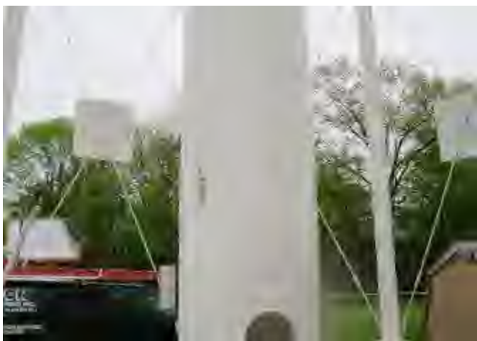
(10) Delaminated coating on riser, and rust staining.
