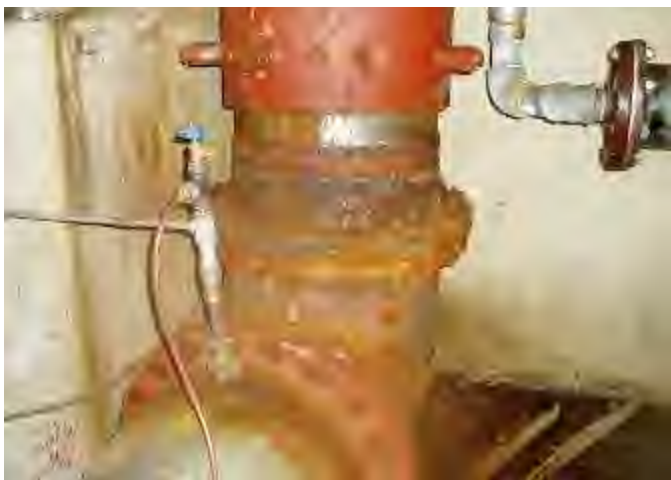
(48) Rusty pit piping and flanges.
