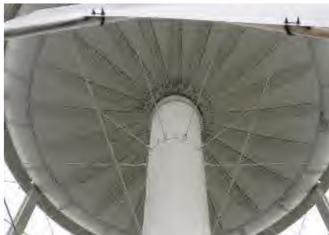
(13) Bottom of bowl, and areas of topcoat delamination.
