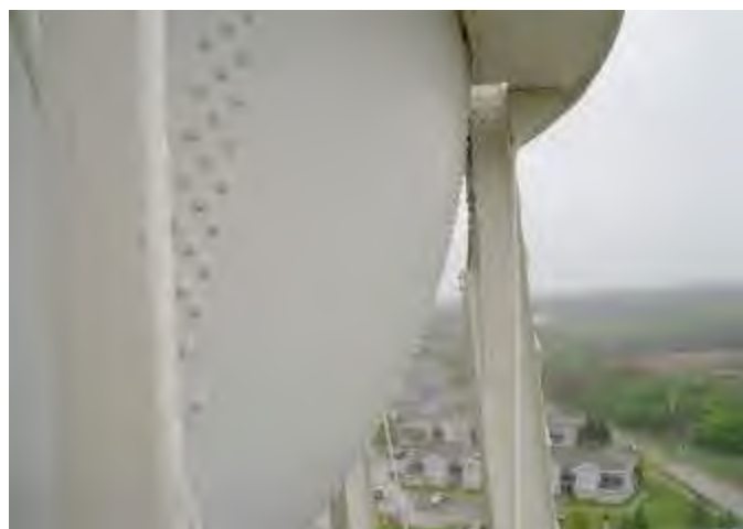
(15) Coating intact on upper bowl.
