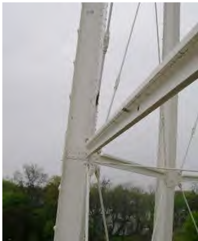
(7) Delaminated topcoat on leg and leg strut.
