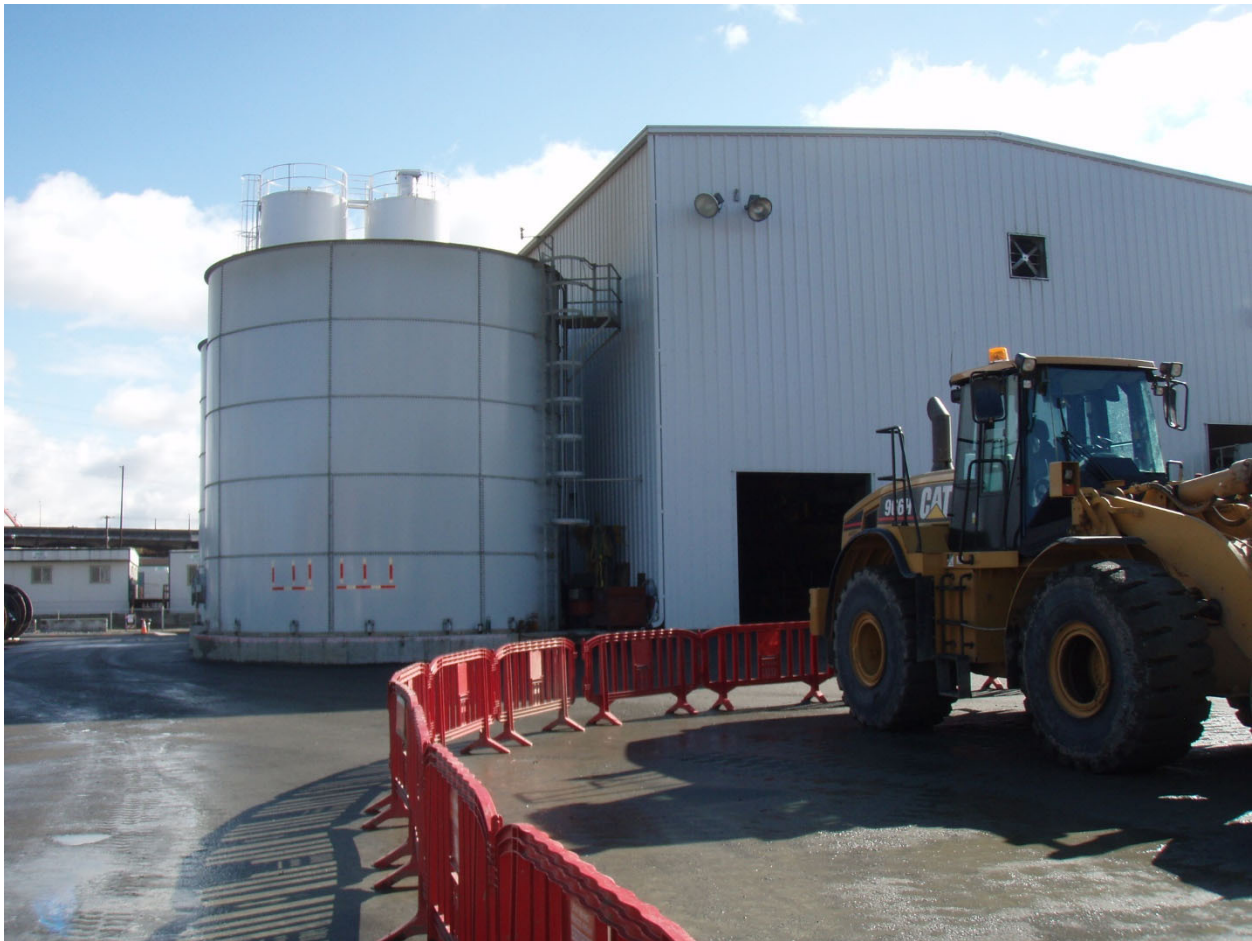
Figure 3. Storage Facility Outside of Slurry Treatment Plant
