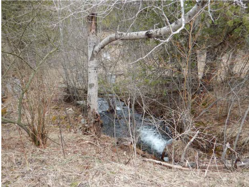
19: Wetland R impoundment culvert outfall to the south
