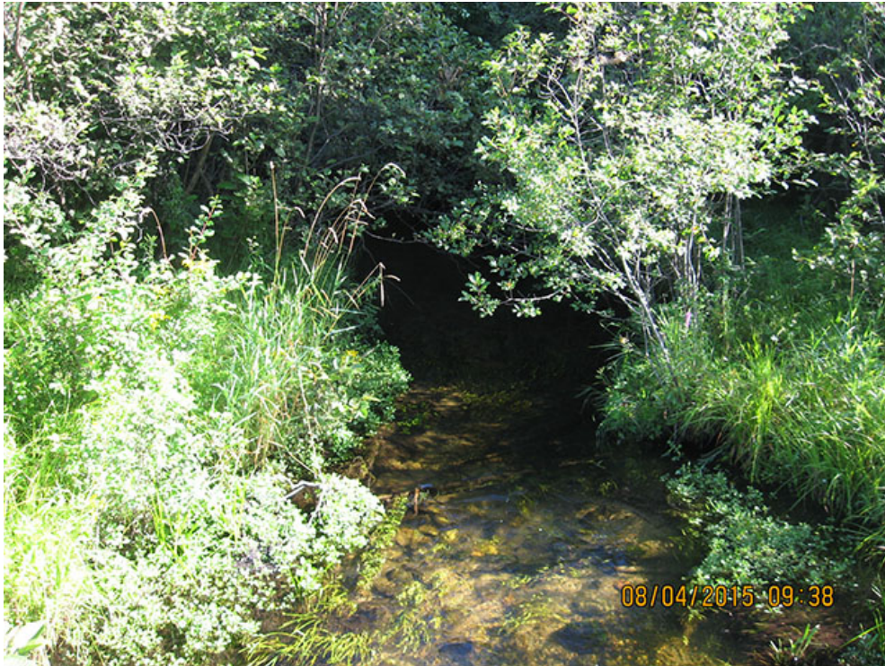
Photograph 7. Station SF 9 – Downstream Extent View Northeast.
