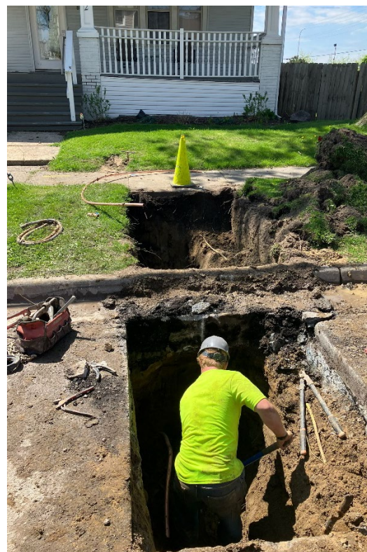
A lead service line is replaced in Ferndale
