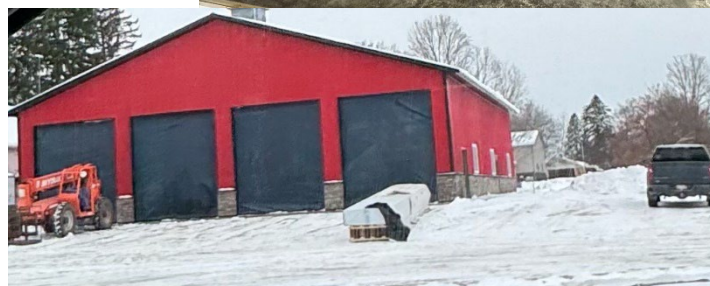
A new barn for fire trucks and equipment in Day Township, Montcalm County.
