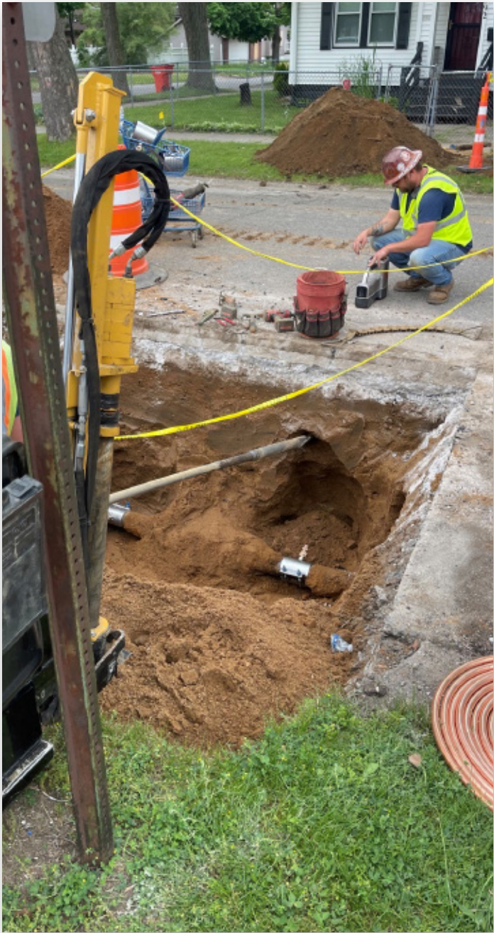
Work crews replace lead drinking water service lines in Benton Harbor in 2022. Photo courtesy of Abonmarche Consulting.
