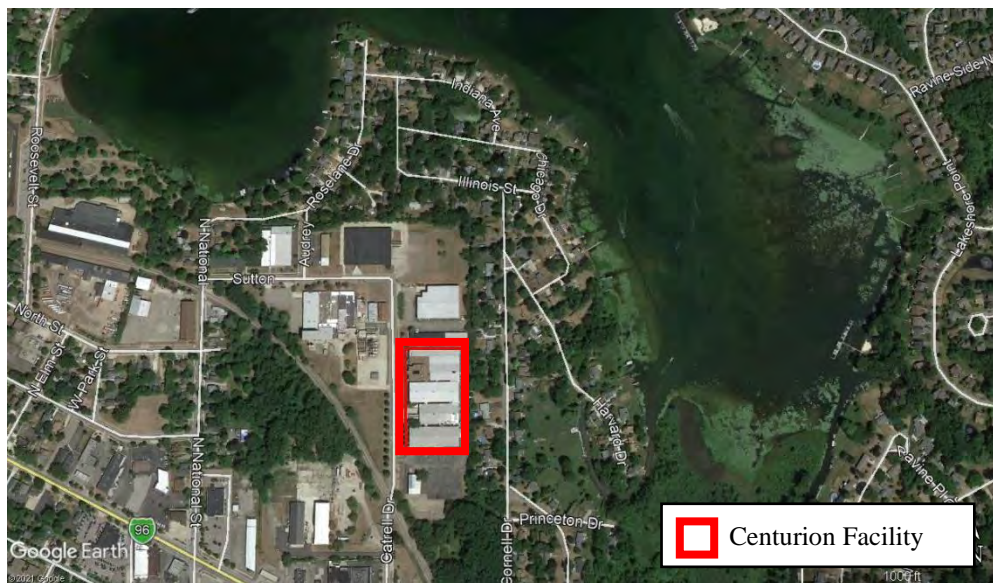
Figure 1. Centurion Medical, Inc. facility located in Howell, Michigan.
