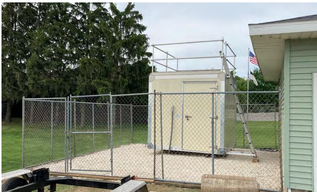
Figure 1.1: Jenison Monitoring Site
