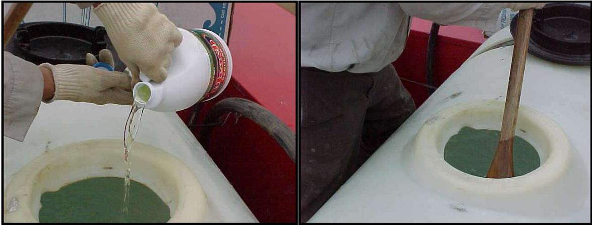
If calcium hypochlorite is used as the source of chlorine, it should be dissolved in a pail of water before being added to the prepared source water. After being added to the bulk tank and thoroughly mixed, the calcium carbonate impurities should be allowed to settle to the bottom of the tank. The clear solution above the sediment is then drawn off for discharge into the water well. Use sodium hypochlorite if the well water has more than 100 ppm dissolved calcium (calcium carbonate).
