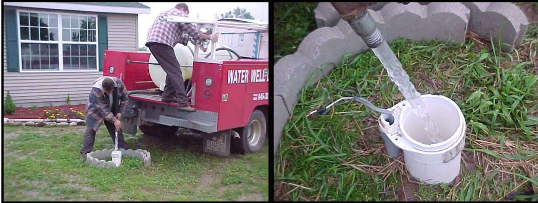
Assure that the wellhead area is well ventilated, especially if the well is in a confined space such as a well house, well pit, or basement offset. Use appropriate safety precautions and follow state laws when working in confined spaces.
