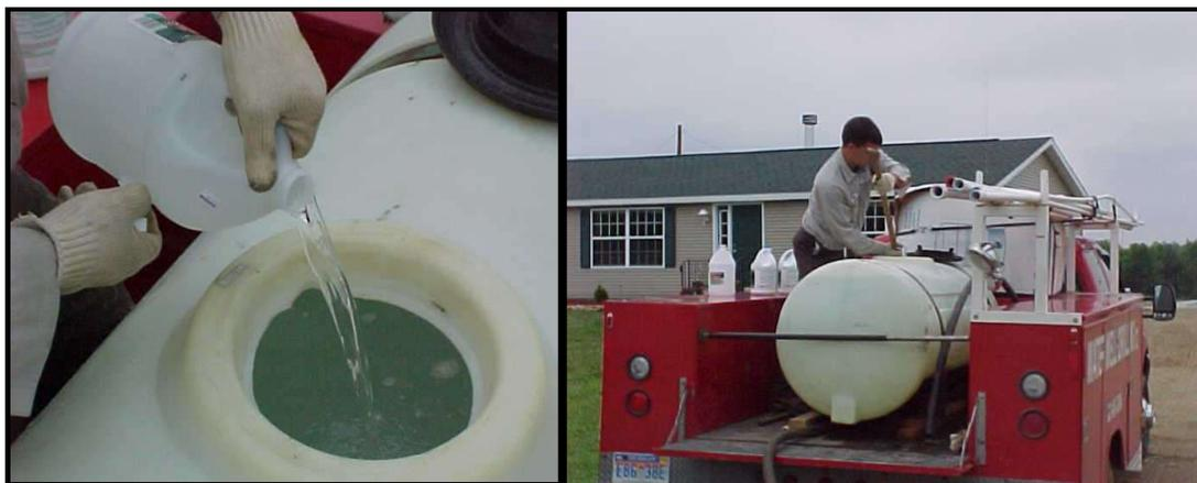
Use a well cleaning acid (carefully following manufacturers' instructions) to lower the pH of the chlorine solution being prepared in the bulk tank to 4 to 4.5. After the acid is added to the water in the bulk tank, the water must be agitated to assure uniform distribution of the acid. An air line, a recirculating pump, paddles, or other agitation methods should be used.
