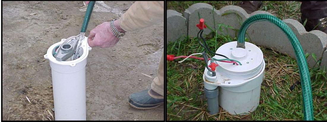
Some water well drilling contractors have extended the recirculation time to several hours. Extended recirculation has been shown to increase the effectiveness of the disinfection process. During extended recirculation a seal needs to be placed on the wellhead to keep contaminants from entering the well.
