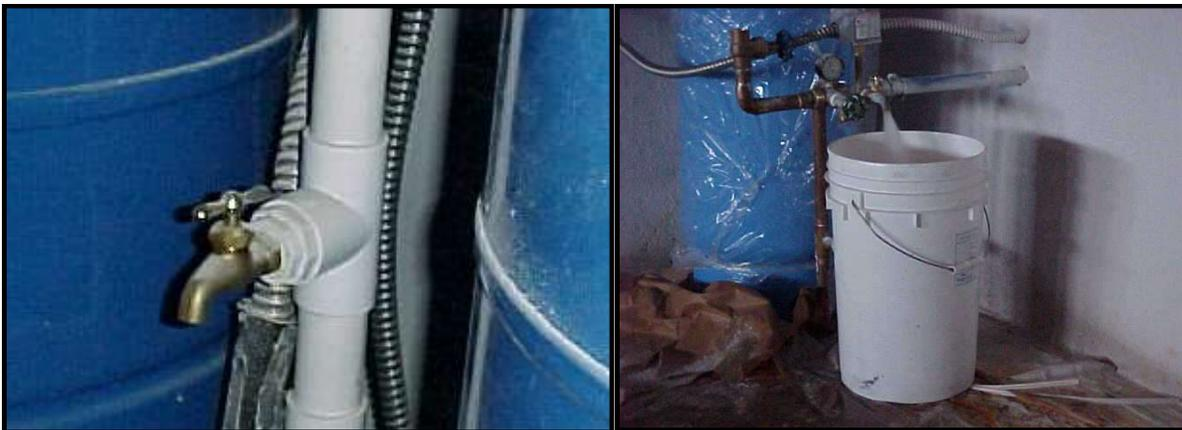
2. Use a smooth bore sampling tap. This allows for a uniform stream of water.
