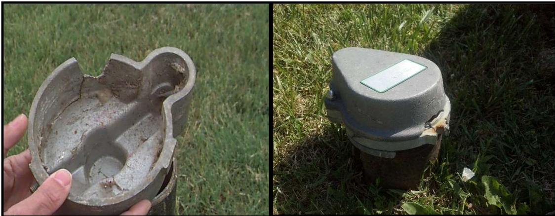
4. **Deteriorated or Damaged Casing.** Any opening in the casing caused by mechanical damage (e.g., hit by snowplow or other vehicle or damaged by vandalism) or corrosion may allow contaminants to enter the well. Damaged casing should be replaced, or the well should be properly plugged and a new well installed.
