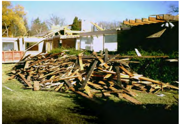
Valuable lumber being salvaged for reuse.
