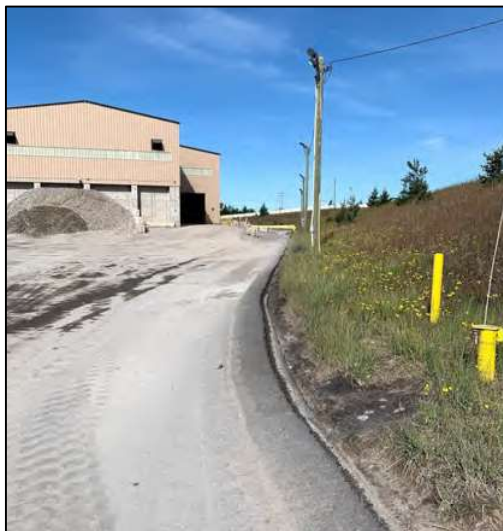
Figure 9 – Curbing Located Near QAL067A
