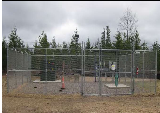
Figure 4 – Domestic Well at the Mine Site
