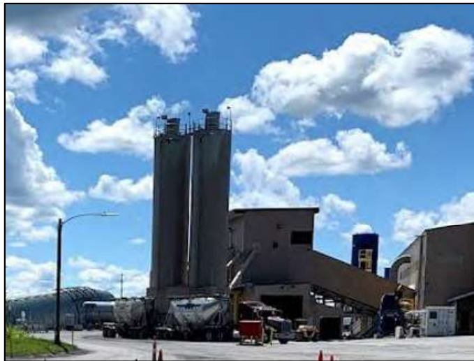
Figure 2 - Cemented Rock Fill (CRF) Plant
