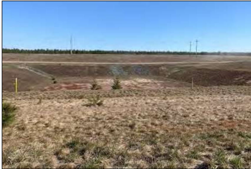
Figure 7 – Non-Contact Water Infiltration Basin (NCWIB) #1 Near the WTP
