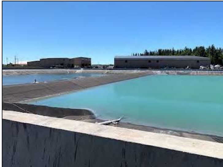
Figure 6 – View looking southeast at CWB #1
