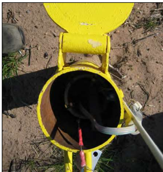
Figure 11 – Piezometer with a Level Troll Located at QAL008A
