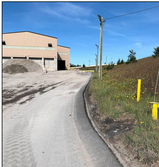
Figure 14 – Curbing Located Near QAL067A
