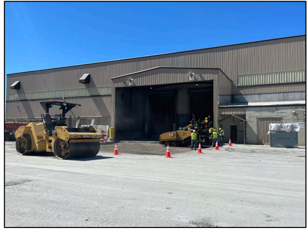
Figure 19 – Paving the COSA Load Bays
