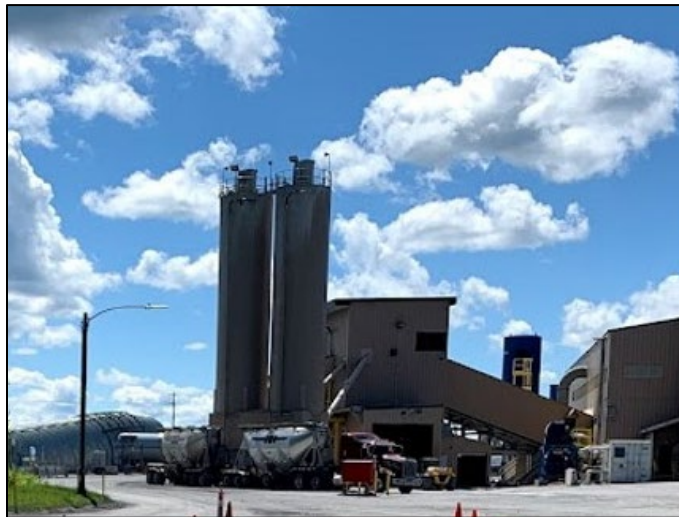
Figure 2 – Cemented Rock Fill (CRF) Plant
