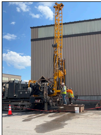
Figure 1 – Drilling Near the Proposed Paste Backfill Project
