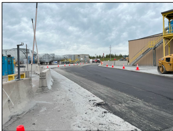
Figure 20 – Paving Between Portal and CRF
