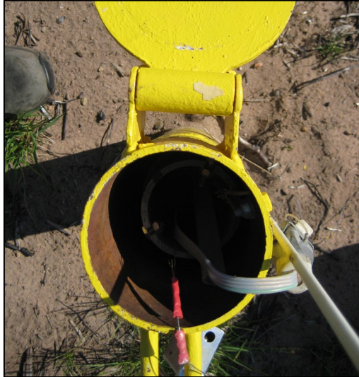
Figure 16 – Piezometer with a Level Troll Located at QAL008A
