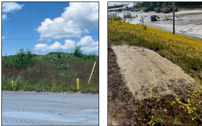
Figure 17 – Hydroseeding on the TDRSA Berm and Additional Mulch
