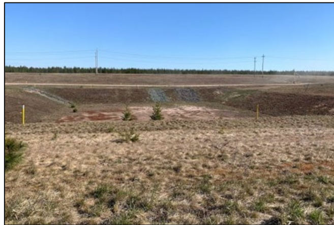
Figure 12 – NCWIB #1 Near the WTP
