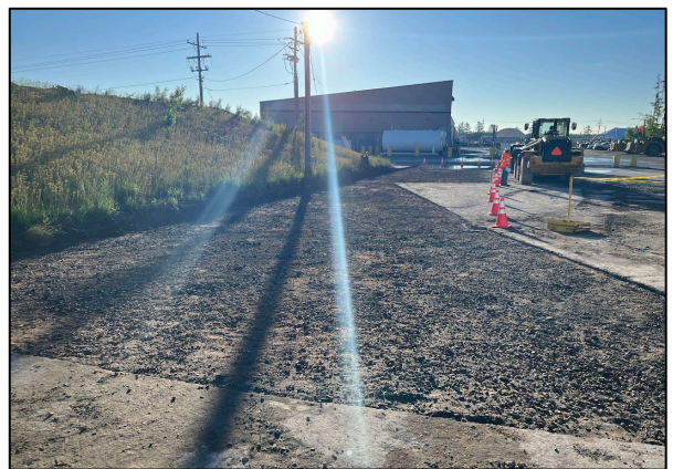
Figure 21 – Paving East of the ASB
