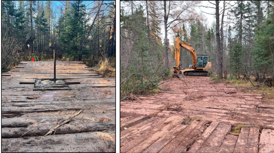
Figure 4 – Installation of two MPBXs above the crown pillar into bedrock
