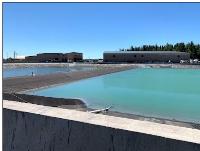
Figure 11 – View looking southeast at CWB #1
