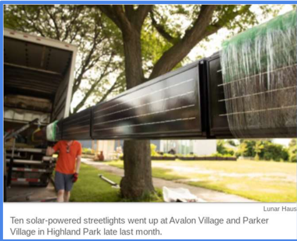
Solar Streetlight Installations
